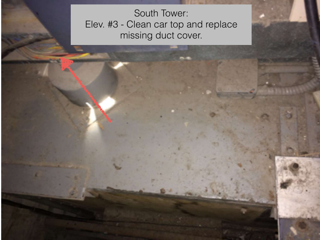
South Tower: Elev. #3 - Car Top debris.
